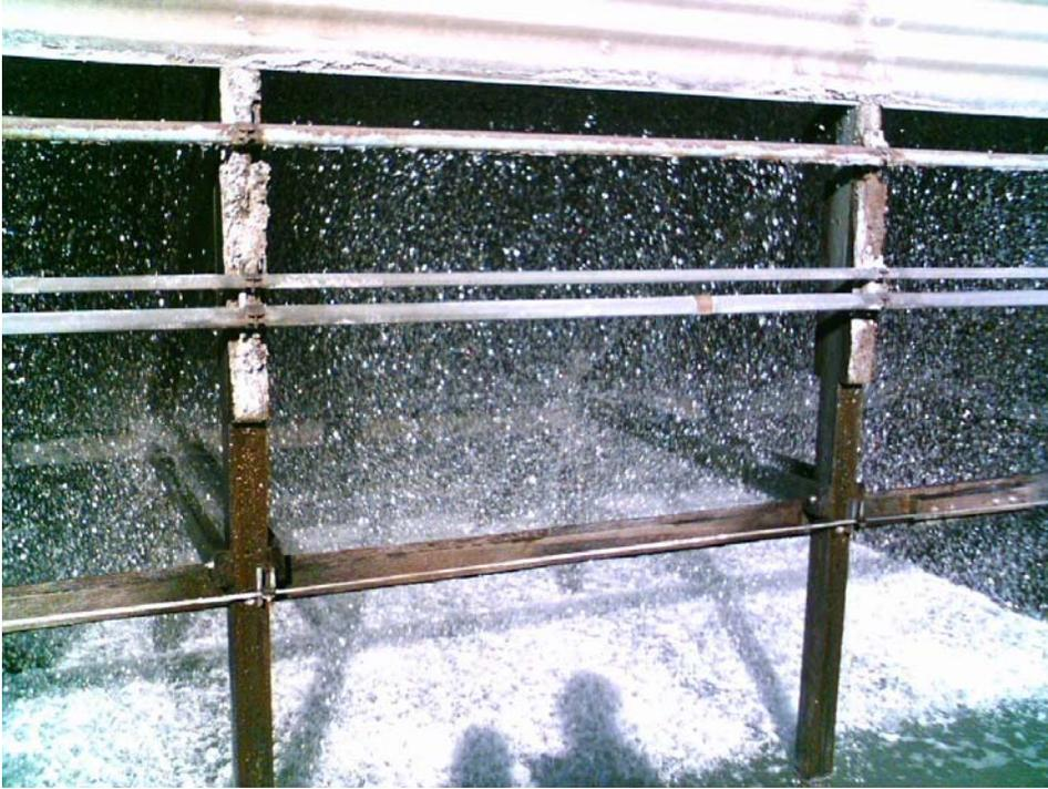
Picture 1: Cooling tower basin and support structure (before), Sep 22, 04
